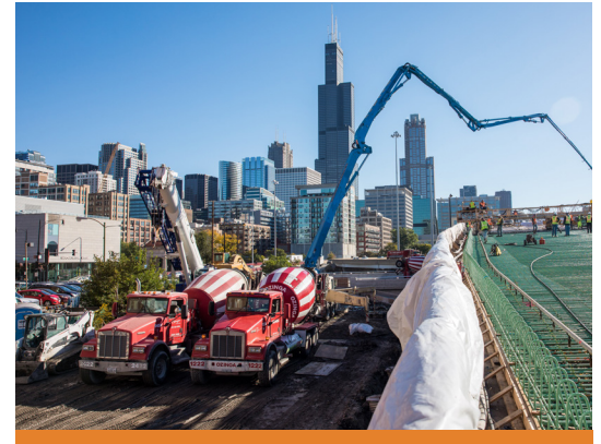
Ozinga Ready Mix has been producing CO 2 mineralized concrete via CarbonCure since 2016.
