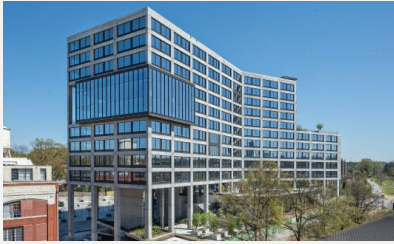
Atlanta, GA – 725 Ponce Concrete Producer: Thomas Concrete CO 2 Saved: 1,500,000 lbs
