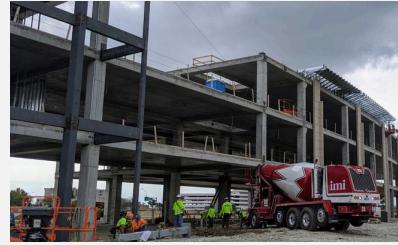
Indianapolis, IN – Infosys Innovation Hub Concrete Producer: Irving Materials CO 2 Saved: 240,000 lbs
