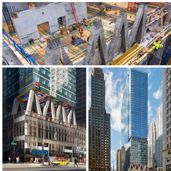
Images of 300 North Michigan Avenue in Chicago.
